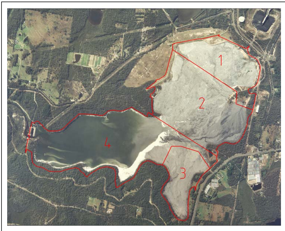
Fig 1 Vales Point ash dam
